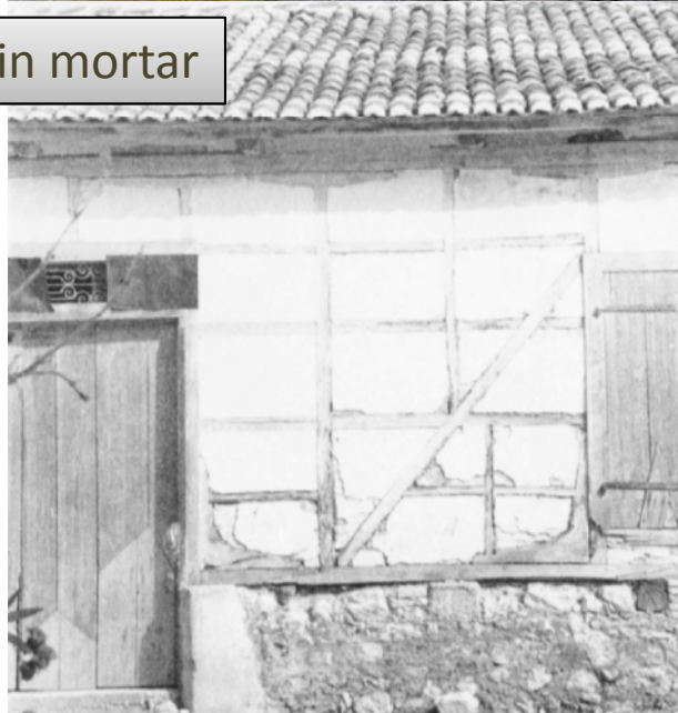
4 th step: separation of diagonals – infill failure
