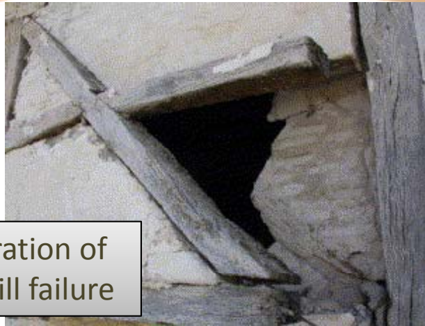
1 st step: cracks in mortar
